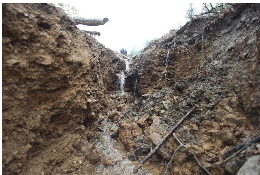
Fig.7 Erosion on skidding tracks in the P. Incurcat area
